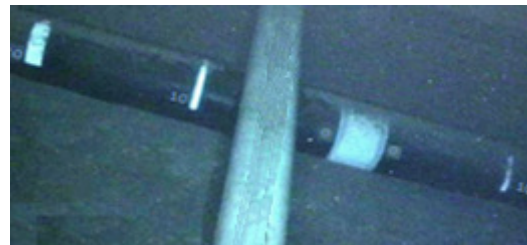
Engineered Lateral Buckle in a Subsea Pipeline
