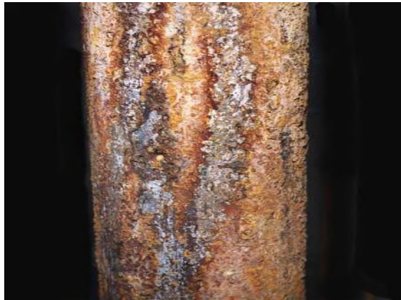
Figure 2 General corrosion of external surface of pipework
